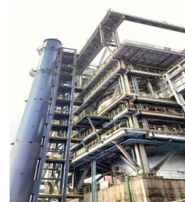
Coke Dry Quenching at Vijayanagar
