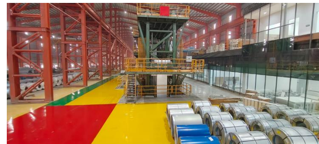
Colour Coating line in Jammu & Kashmir
